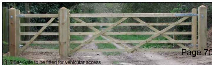
1.5m Bar Gate to be fitted for vehicular access
